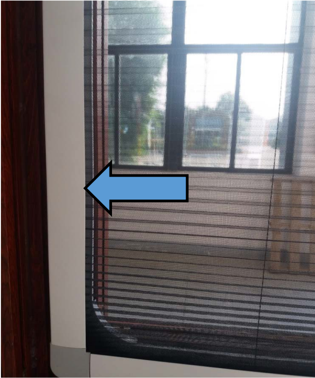
Step 3—Push fastener up to tighten
