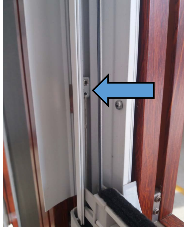
Step 4—Tighten LH & RH fastener evenly
