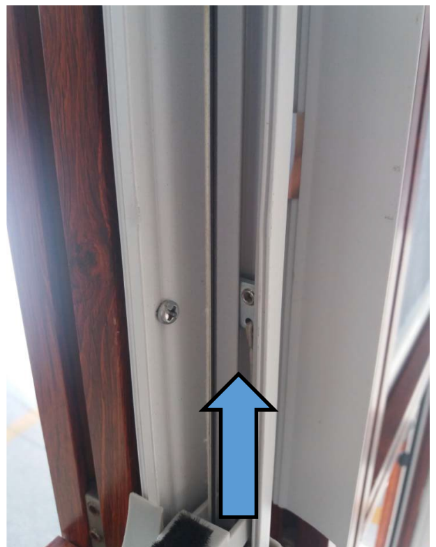
Step 4—Tighten LH & RH fastener evenly
