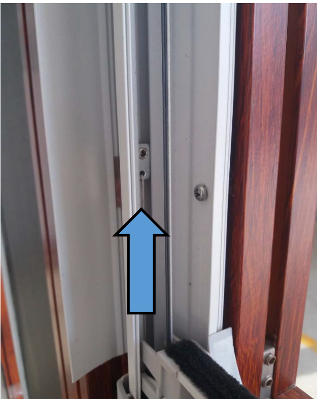
Step 3—Push fastener up to tighten
